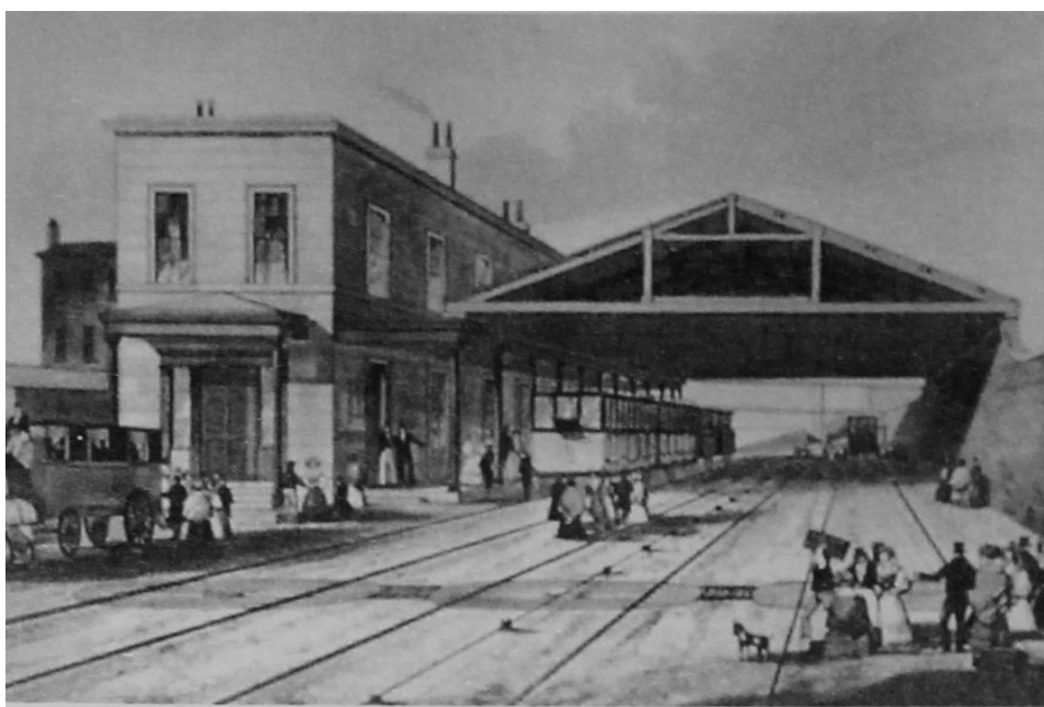
Figura 01. Liverpool - Crown Station, 1830. Fonte: PEVSNER, Nikolaus - A history of building types . London Thames and Hudson, 1997.
